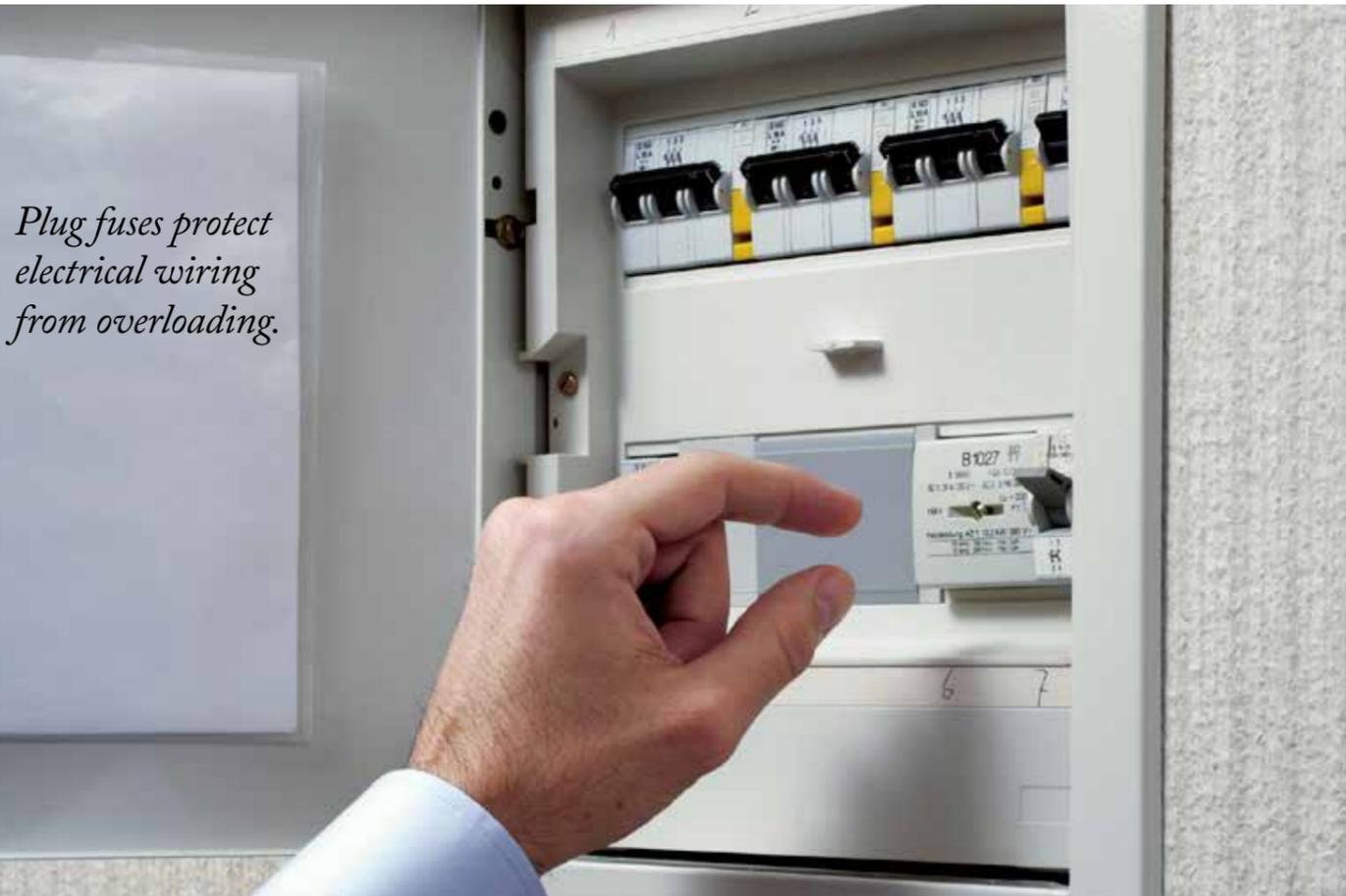
*Plug fuses protect electrical wiring from overloading.*
